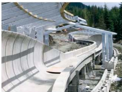
Track sections under construction. Above photos courtesy of Stantec.
